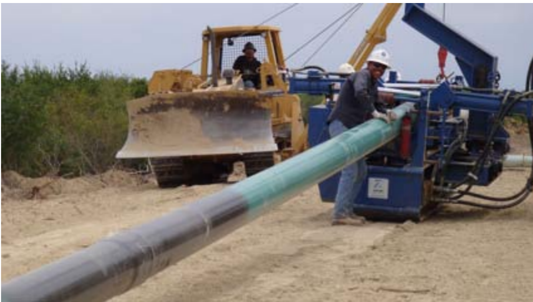
Side-boom installation of coated pipe
