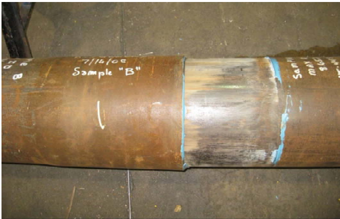
Figure 2: Pressure Containment Loss: Pull-out
