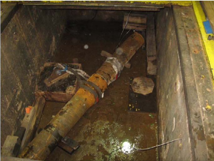
Figure 10: Burst Test Setup for 10" Zap-Lok ® in covered pit
